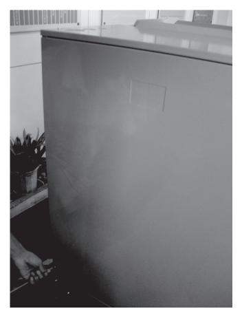
**2.** Remove the cover plate from the air handler.
