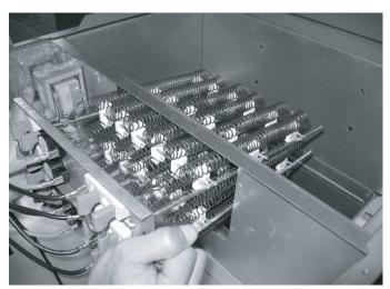
**4.** Align the attachment clip and the hole and fasten the loose wires by using wore tie.
