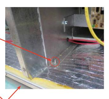
**6.** The last screw to remove is located on the inside back panel visible above the inducer assembly.
